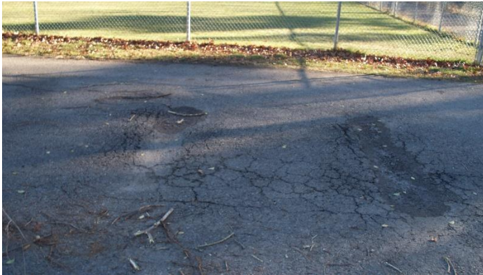
Damage to asphalt from weight of trash truck
