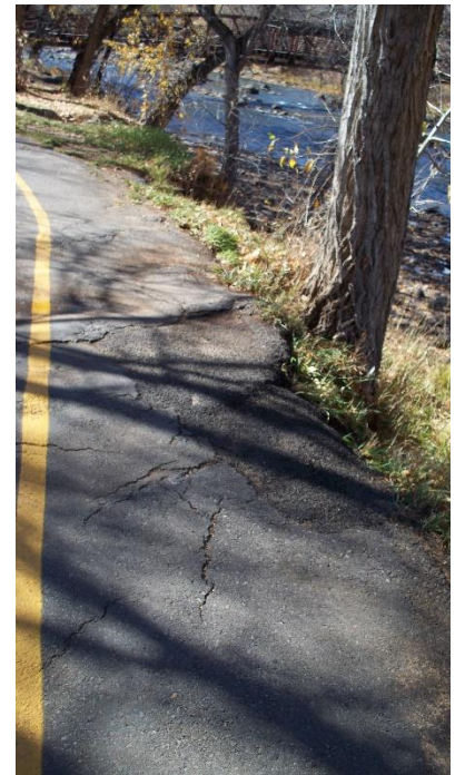
Heaving section of the trail
