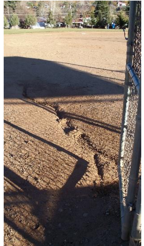
Erosion at dugout entrance
