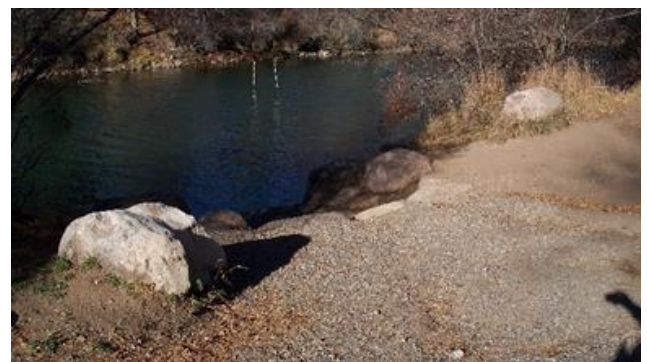
Example of rock armoring of river bank
