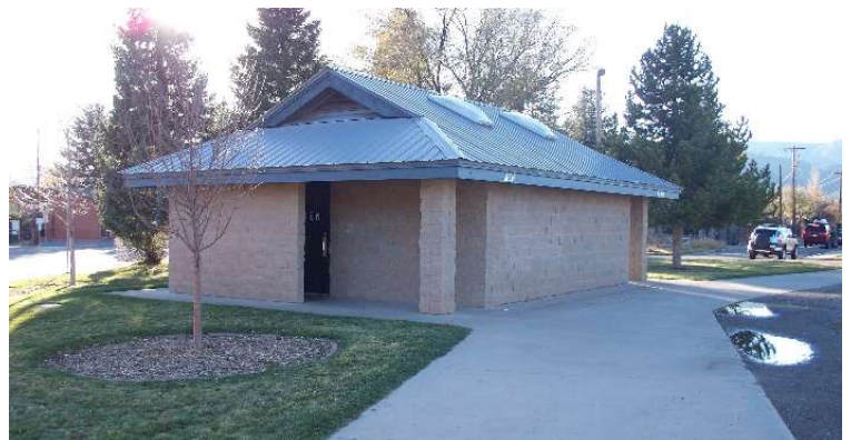
Restrooms at Riverview Sports Complex
