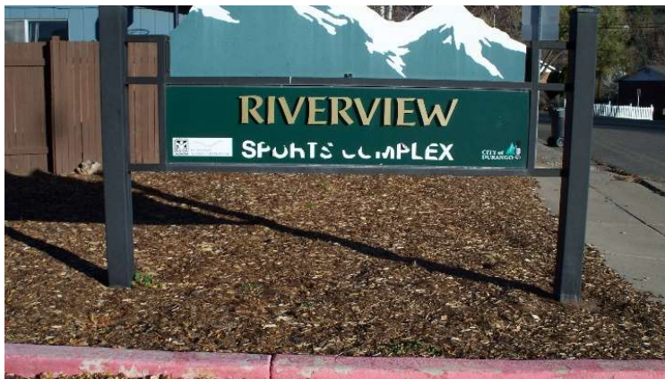
Example of peeling letters on park sign
