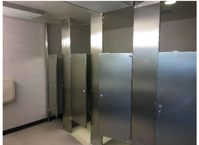
Newly renovated restrooms at Durango Softball Complex
