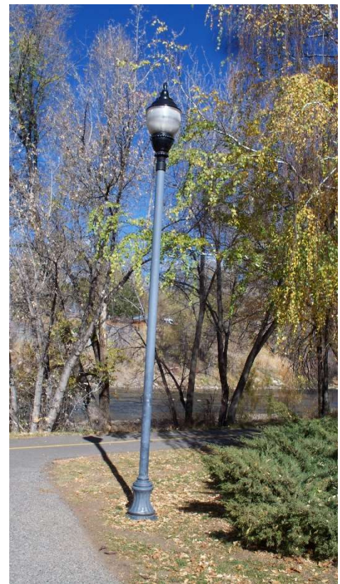
Trail lighting in Iris Park
