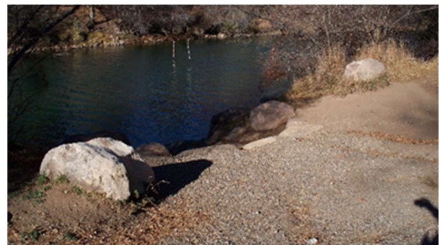
Example of rock armoring of river bank
