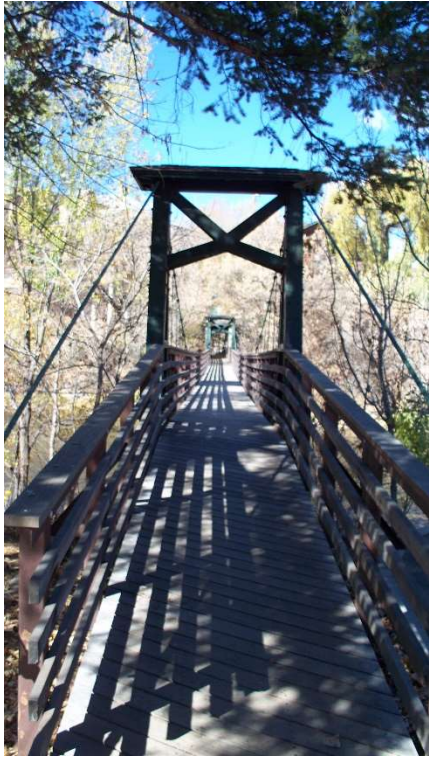
Bridge over the Animas River
