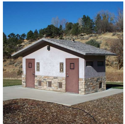
Restroom facility at Jenkins Ranch Park
